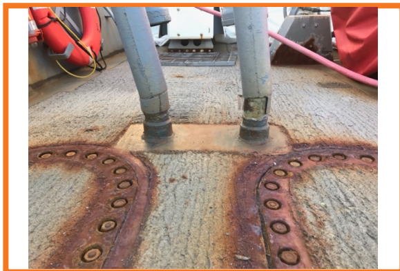
Kick Pipes Prior To Coating
