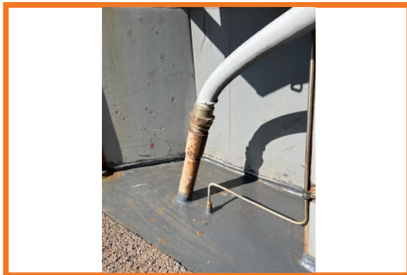
Kick Pipe Prior To Coating
