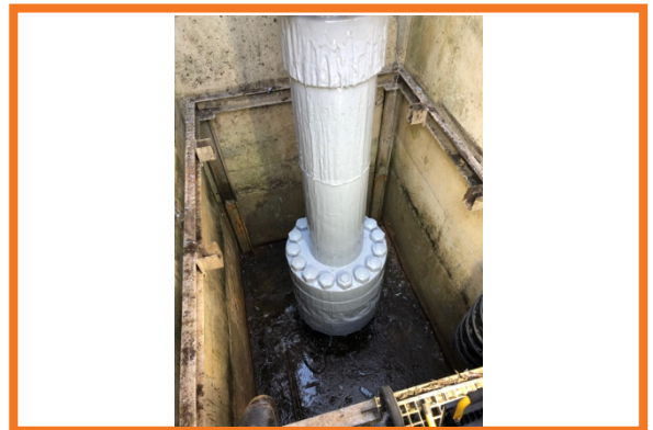
Lower section of wellhead complete
