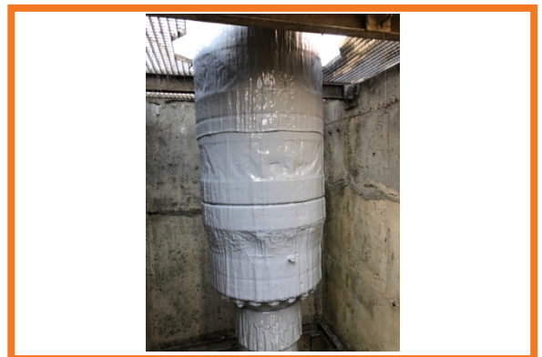
Completed section of wellhead
