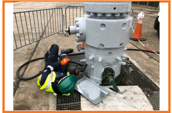
Oxifree TM198 application taking place
