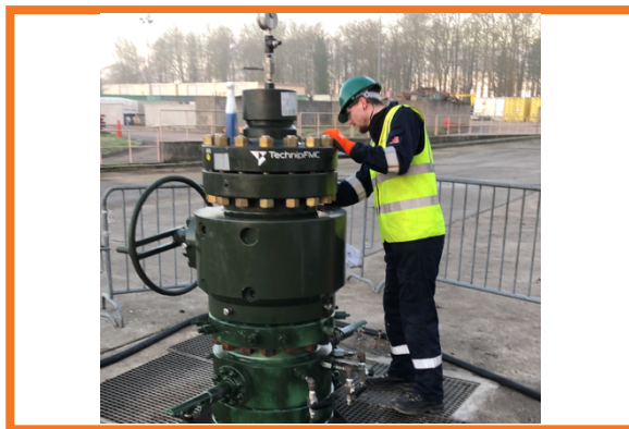
Carrying out minimal surface preparation
