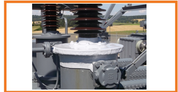
Application of repair bandage
