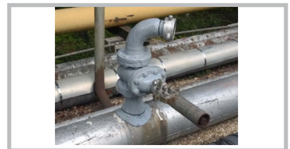
Hydrant after TM198 application
