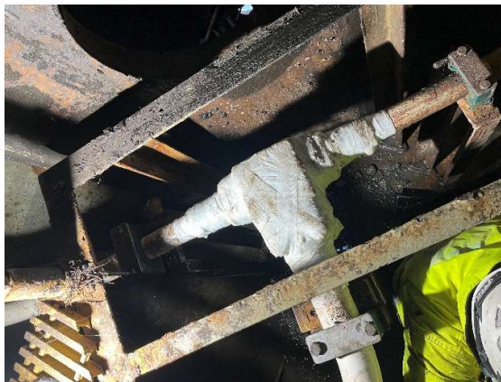
Block covered with Oxitape above TM198
