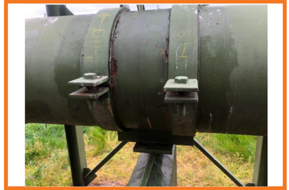
Pipe Clamp Assembly Encapsulated by Oxifree TM198
