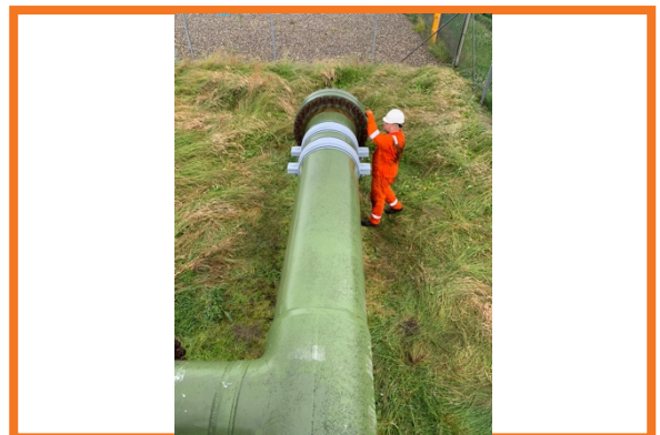
Pipe Clamp Assembly Encapsulated by Oxifree TM198
