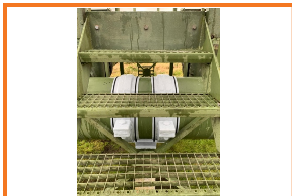
Pipe Clamp Assembly Encapsulated by Oxifree TM198
