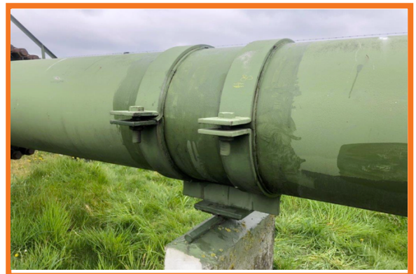
Pipe Clamp Assembly Encapsulated by Oxifree TM198
