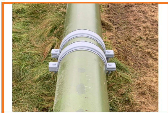
Pipe Clamp Assembly Encapsulated by Oxifree TM198
