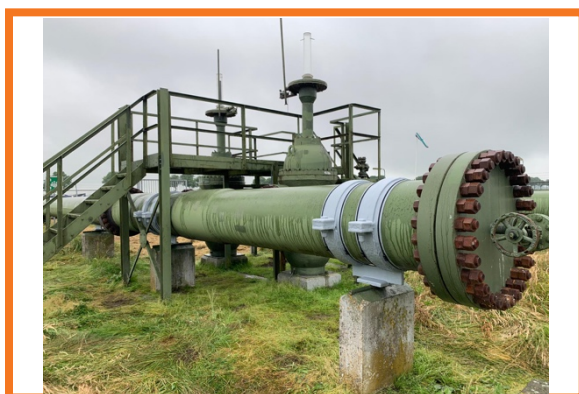
Pipe Clamp Assembly Encapsulated by Oxifree TM198
