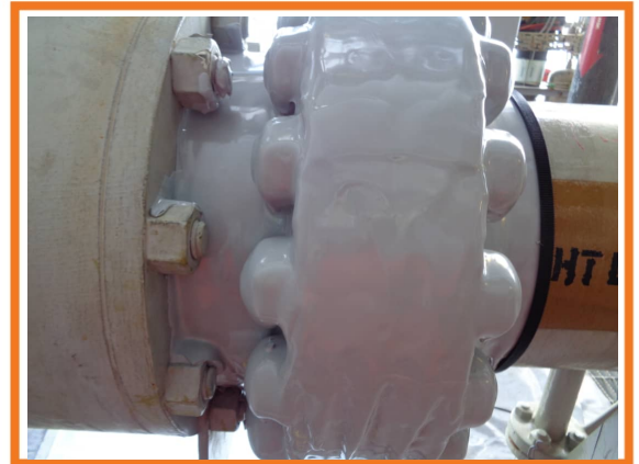
Pictures of the substrates with Oxifree TM198 after job completion
