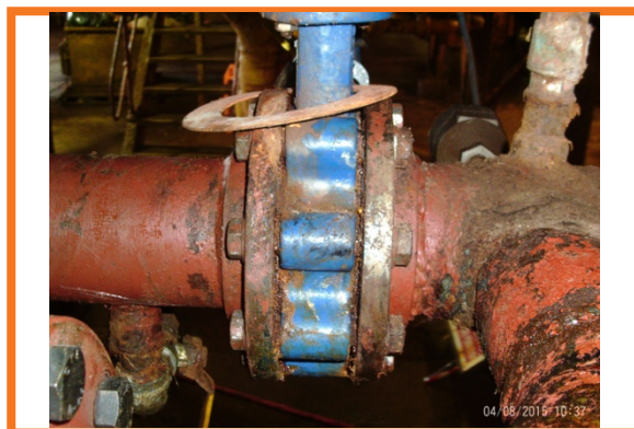
Flanges & Valve Prior To Coating
