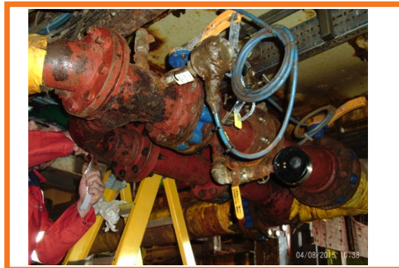
Flanges & Valve Prior To Coating
