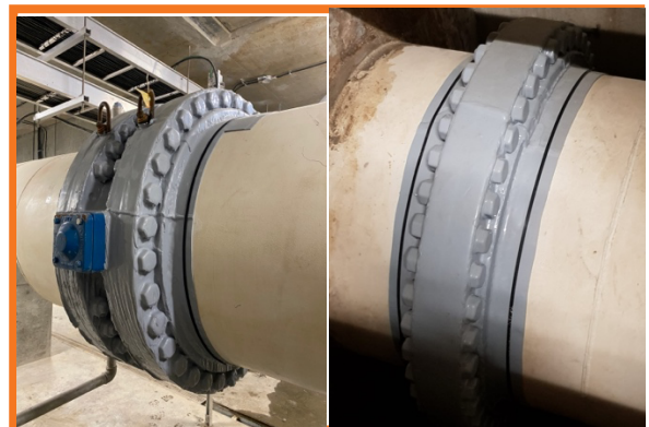
Completed Flange Assemblies
