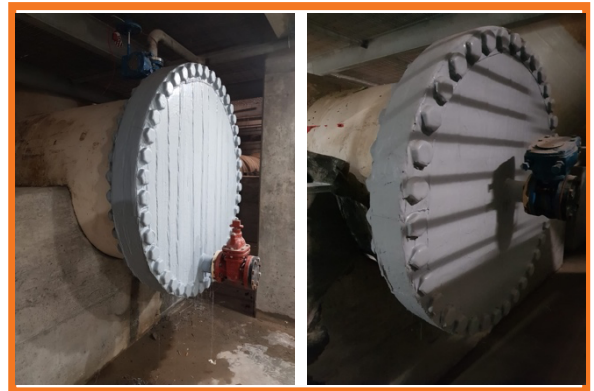
Completed Blind Flanges
