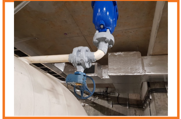
Completed 4" Flange Assemblies
