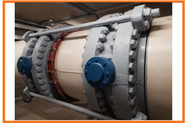
Completed 54" Coupling Assembly
