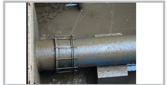
Pipe coupling prior to clean and application
