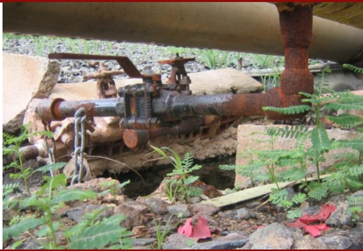
Gate valves with varying corrosion damage to almost all surfaces
