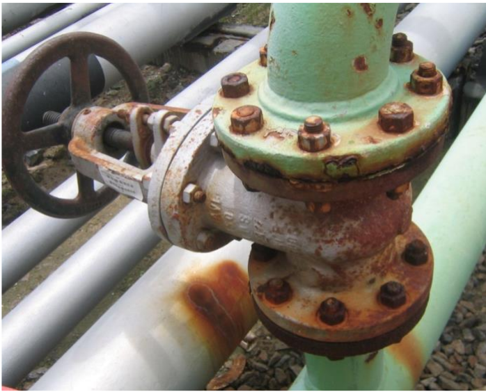
Gate valves with varying corrosion damage to almost all surfaces
